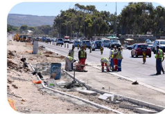
Road Network Rehabilitation
