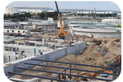
Potsdam WWTW Upgrade
